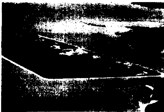
Figure 7. Grassy Island, a diked containment structure for harbor dredgings in Toledo Harbor, Ohio. Note marsh formed inside the dikes (May 1966).
