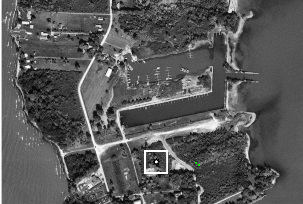
Figure 1. Location of the artificial hibernation structures on Middle Bass Island State Park property.
