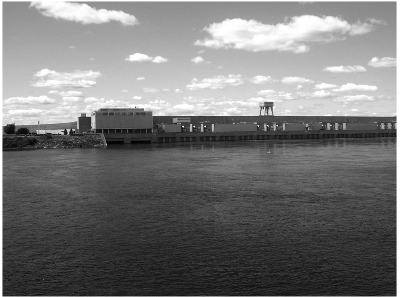
The Moses-Saunders Dam: Photo Courtesy of Dalton Foster
