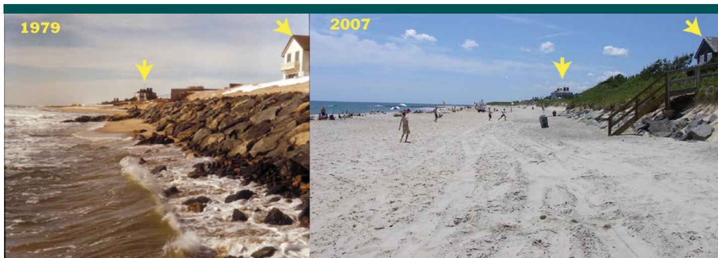
Figure 24. In stable areas with an adequate sand supply, studies over the last thirty years have shown shore parallel structures like this rock revetment can provide erosion protection during severe storms without adversely affecting natural beach building processes. (Arrows indicate the same houses in the two photos for reference.) (2007 Photo: M. Slattery)
