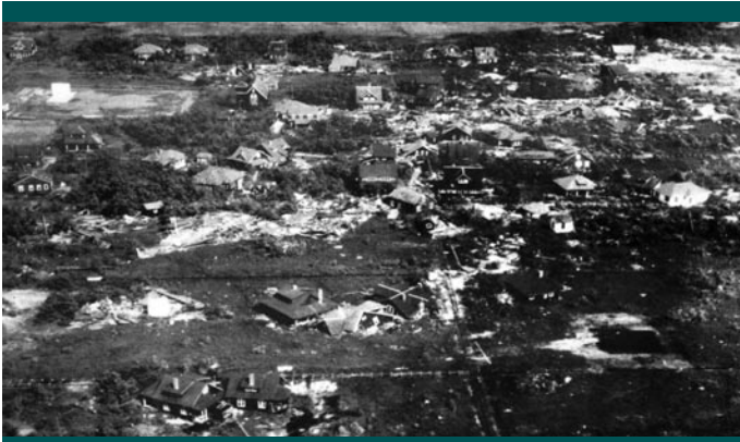
Figure 7. Damage in Saltaire, Fire Island, caused by the 1938 hurricane. (Photo: U.S. Army Corps of Engineers 1958)
