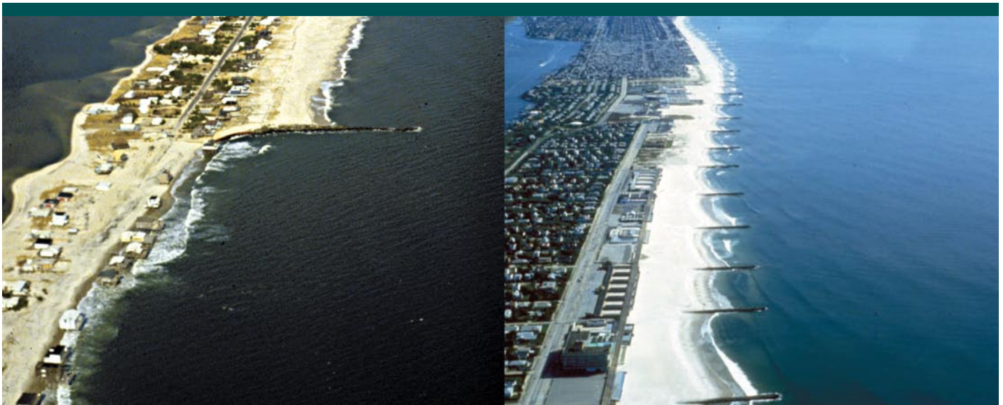
Figure 23. Groins interrupt the natural flow of sand and can increase erosion in adjacent areas (left). However, these structures can be designed to slow down erosion and minimize adverse impacts in certain situations. The 49 groins constructed in the 1920s in Long Beach (right) have helped maintain a recreational beach that protects the developed upland.
