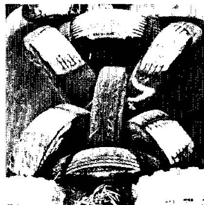
Figure 24. Supplemental buoyancy is highly desirable in areas having heavy winter snowfall or marine fouling organisms. Note submerged tires in this FTB section.
