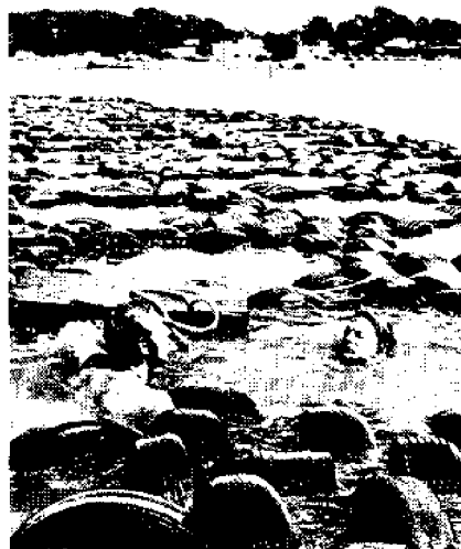
Figure 34. Divers bind adjacent sections together to construct the FTB.
