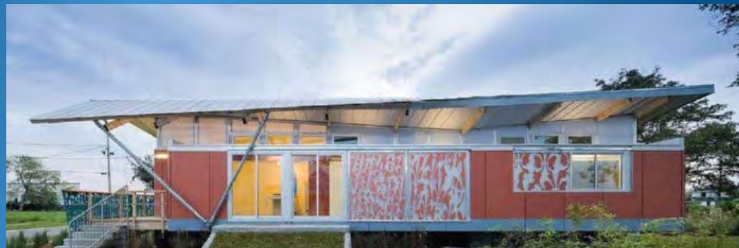
Flat House, designed by Morphosis Architects and students from UCLA collects its rainwater and generates its own electricity and is capable of floating as high as 12-feet on rising waters. www.makeitrightnola.org Pic by [unclear] aan
