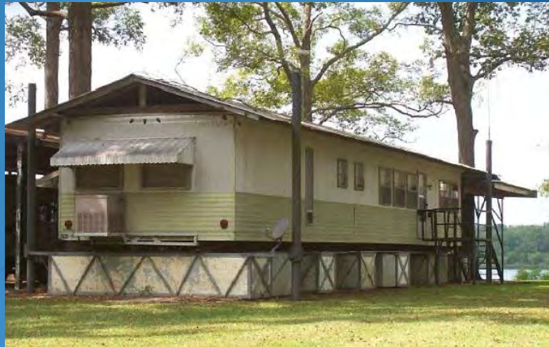
On the Mississippi, the easiest homemade solution, foam blocks under your home. The 4 guide posts keep the house in place as it rises, just like a floating dock. www.buoyantfoundation.org
