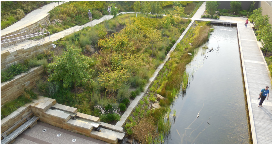
This constructed wetland and pond is part of the Phipps Conservatory's LEED Platinum® Center for Sustainable Landscapes (CSL).
