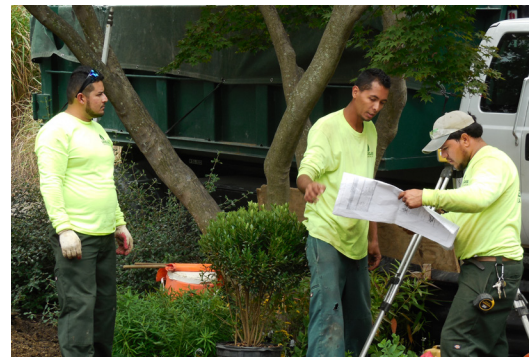
A well-prepared crew consults a full-size printed drawing during plant installation.
