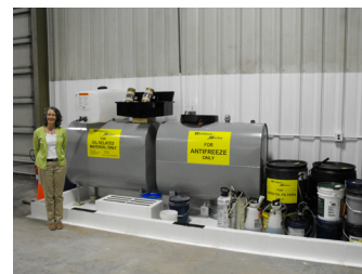
Waste containers and containment at Washburn Marina. Photo credit: Gene Clark, UW Sea Grant Institute.
