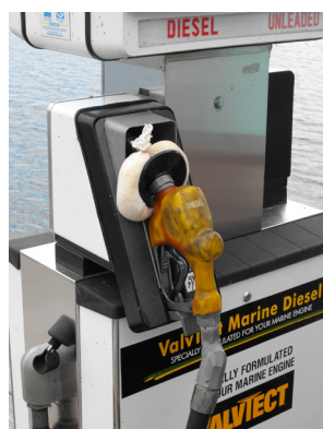
Absorbent pad on fuel pump at Pikes Bay marina. Photo credit: Gene Clark, UW Sea Grant Institute.
