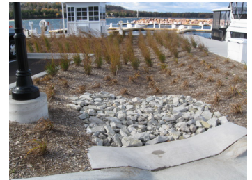
Bio-retention swale at Egg Harbor Marina. Photo credit: Todd Breiby, Wisconsin Coastal Management.
