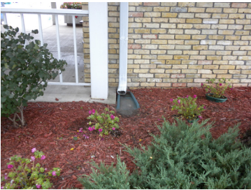
Downspouts at Port Washington Marina. Photo credit: Kae DonLevy.
