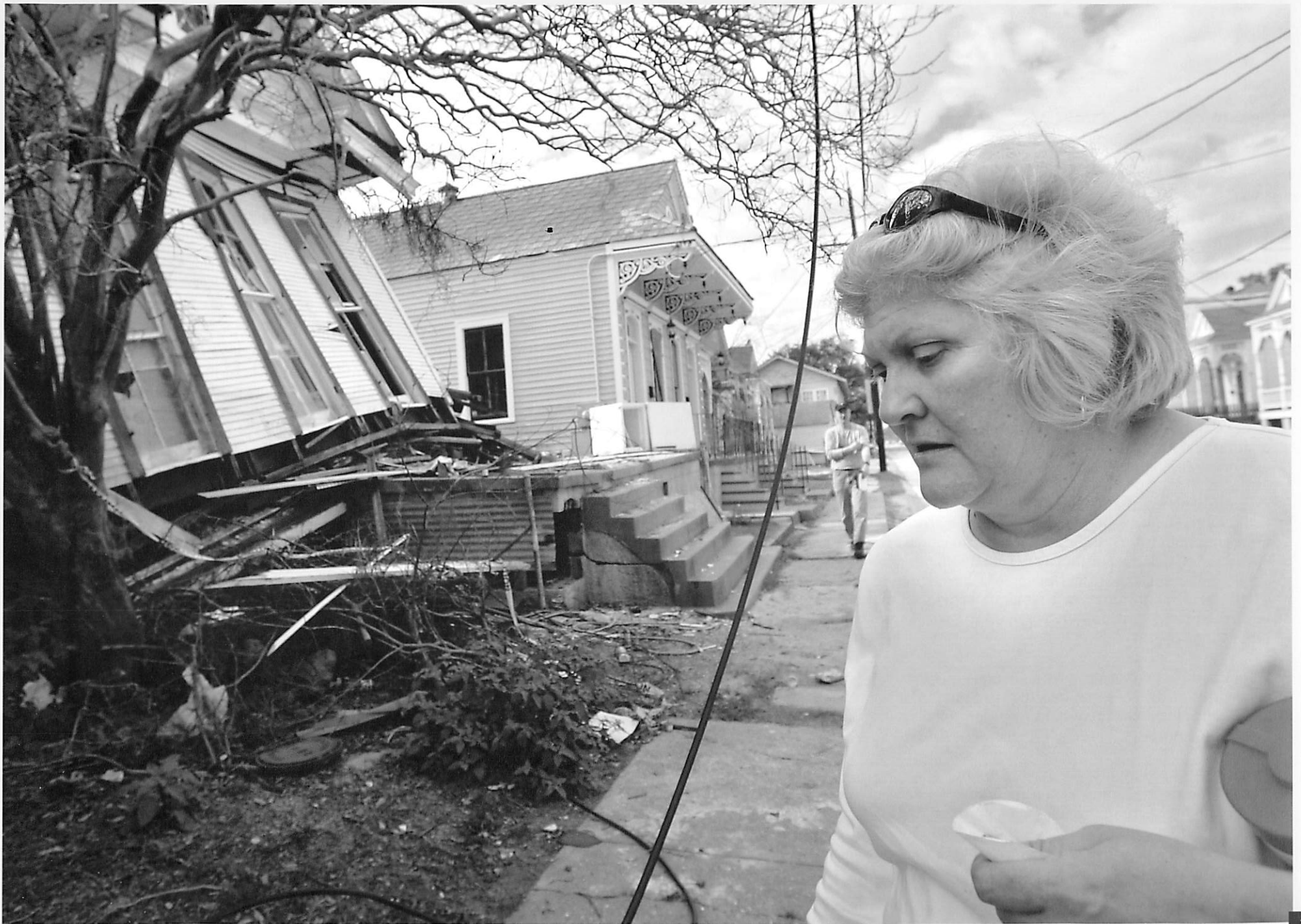
OPPOSITE: This home, 200 yards from the Mississippi coast, survived Katrina's storm surge because its first occupied floor was raised, preserving the elevated living area. PHOTO/Wade Spees ABOVE: New Orleans native and preservationist Stephanie Bruno inspects a house that Hurricane Katrina knocked off its foundation. PHOTO/Wade Spees
