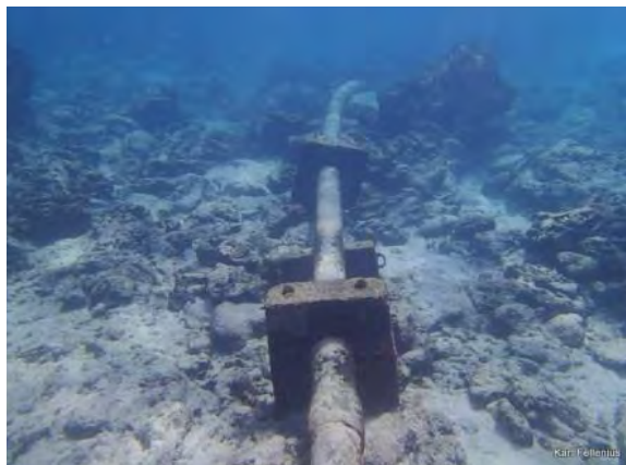
Fig. 4.2.47 Bairiki 23m south of point 18, looking South, corrected depth 1.4m
