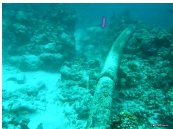
Fig. 4.3.44 From Bikenibeu 34m South of end of existing pipe, looking North, route along ↓ corrected depth 1.7m
