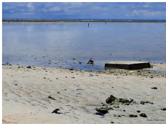
Fig. 2.5 From Betio outfall location, looking South along the existing outfall route
