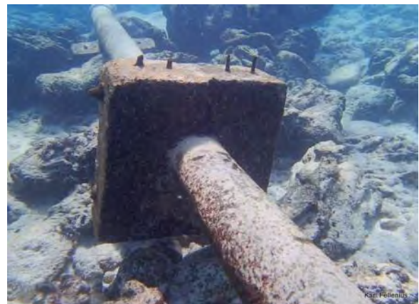
Fig. 4.2.48 Bairiki 26m south of point 18, looking South, corrected depth 1.4m
