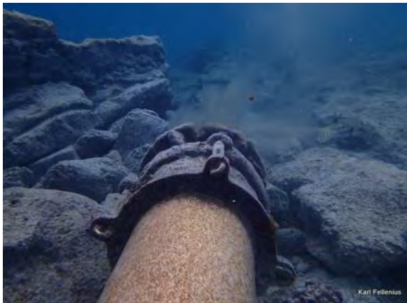
Fig. 4.1.72 From Betio end of existing pipe, looking South, corrected height +0.8m
