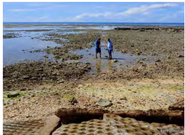
Fig. 2.10 From Bairiki outfall location, looking South along the existing outfall route
