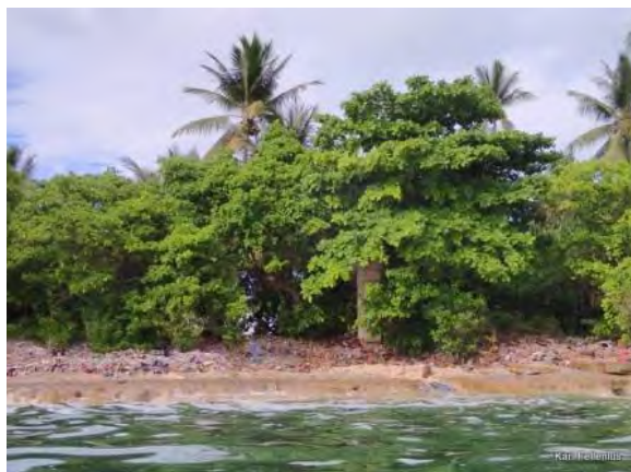
Fig. 2.14 From south of Bikenibeu outfall vent, looking north along the existing outfall route
