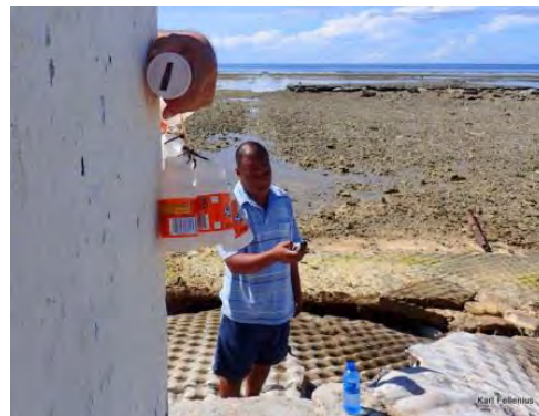
Fig. 4.2.4 Bairiki vent looking South
