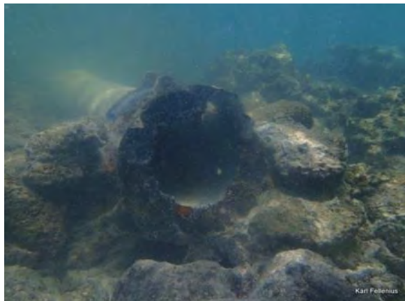
Fig. 4.3.38 From Bikenibeu end of existing pipe, looking Northeast, corrected height +0.3m
