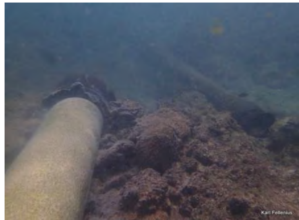
Fig. 4.3.39 From Bikenibeu end of existing pipe, looking South, corrected height +0.3m
