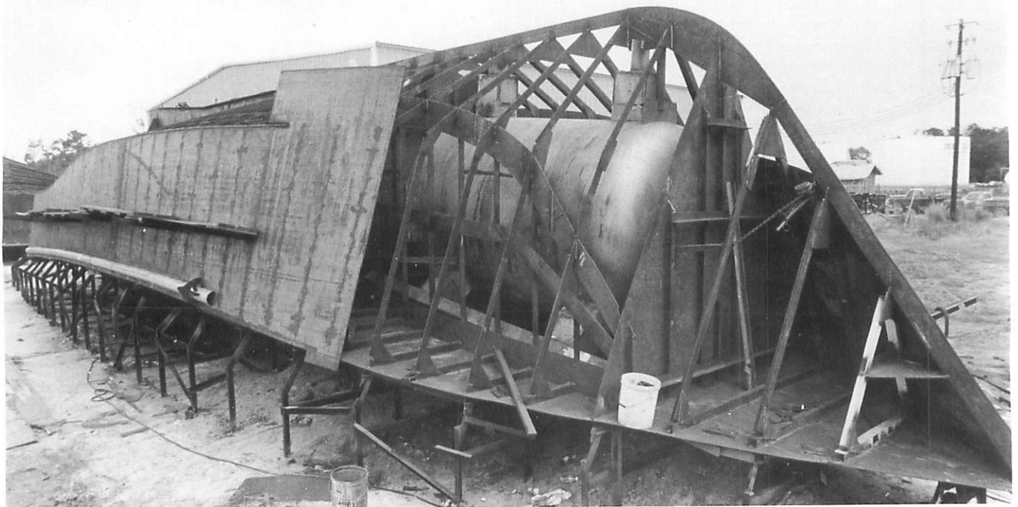
Left: Sea Grant researcher C. Everett Brett of the University of Alabama examines the heads of specially designed cryogenic tanks for storing super cold LNG (liquefied natural gas) on board a new breed of shrimp boat that could cut 45 percent off Gulf of Mexico shrimpers' annual operating costs. Right: Workers prepare for pouring high density foam mounts for the completed tanks. Below: The larger of the two tanks is installed in the vessel's forepeak.
