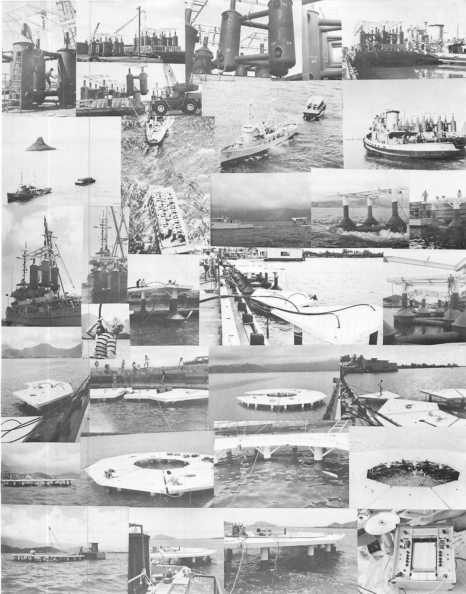
1:20 scale model disassembly, transport to Kaneohe Bay, reassembly "at sea," and initial testing--May, June and July 1972.
