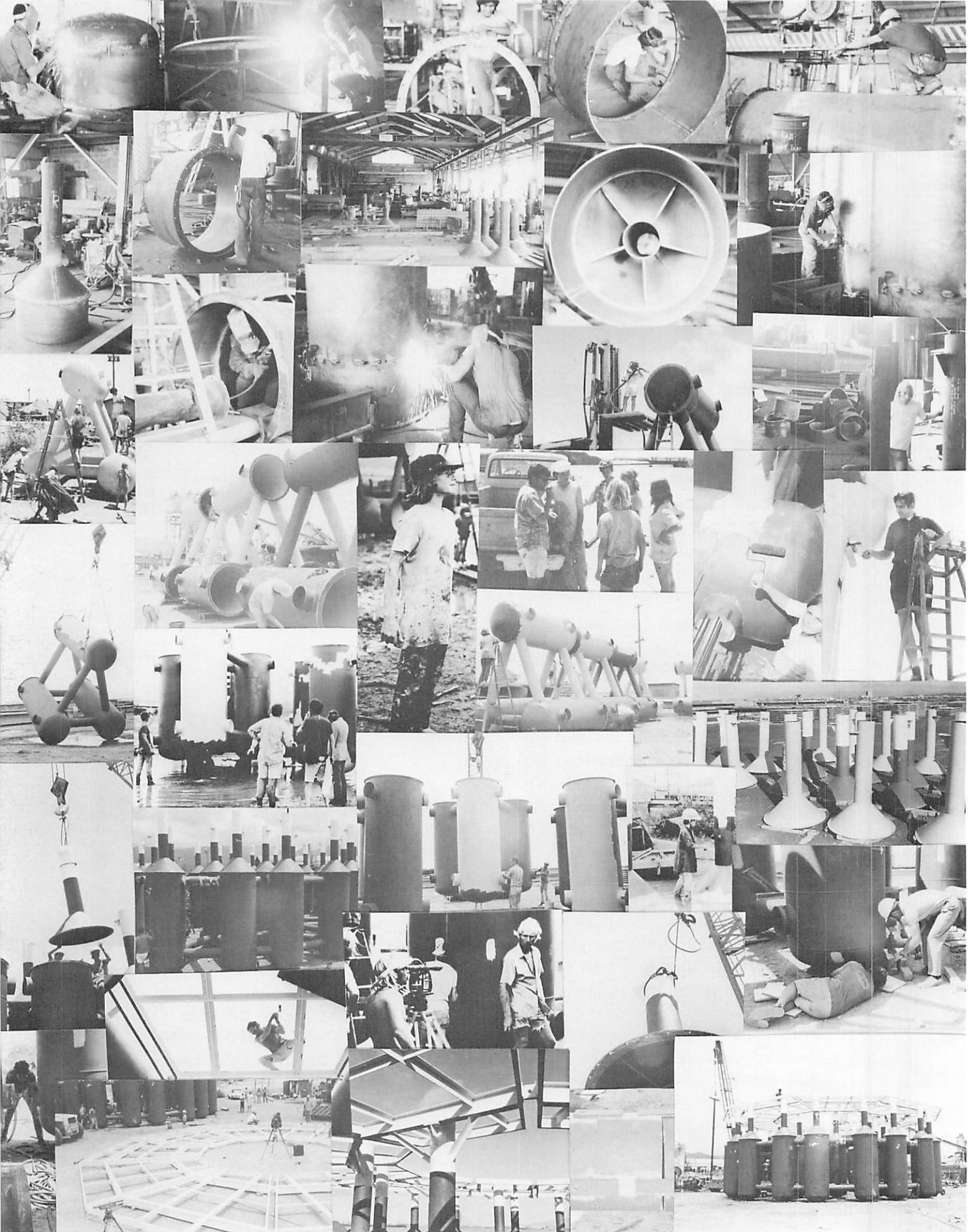
Construction, finishing and pre-assembly of the 1:20 core-ring scale model in the Sand Island industrial district of Oahu--February, March, and April 1972.
