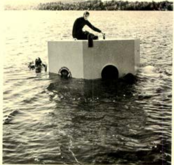
The LAKELAB underwater habitat being placed in Grand Traverse Bay.
