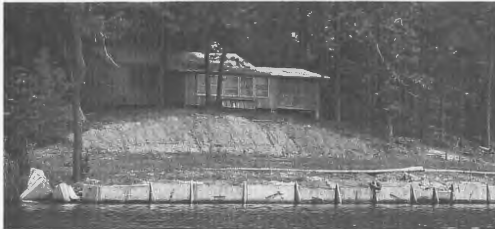
Photo: Bulkheading to slow the inevitable erosion of North Carolina's estuarine shoreline
