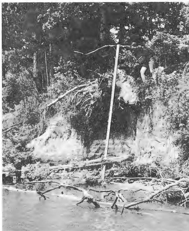
High bank erosion
