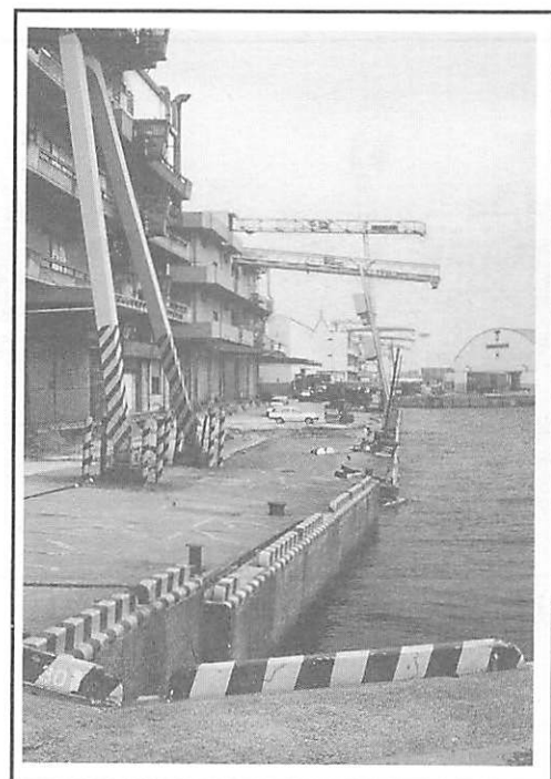
d) Area Between Piers 1 and 2
