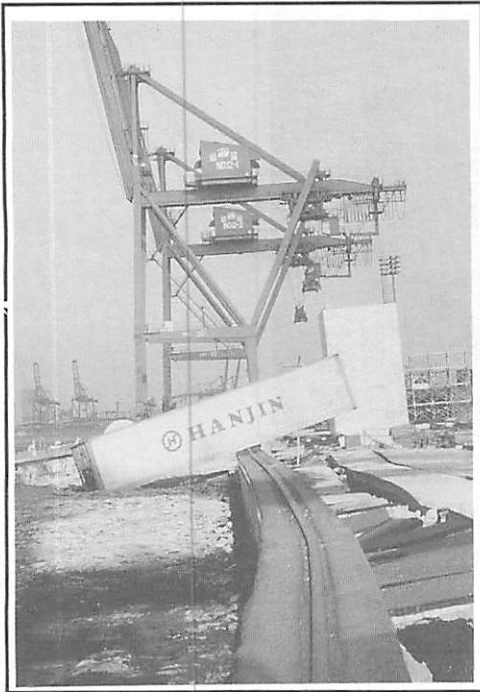
e) Damaged Crane Rail at Minami Wharf, Port Island
