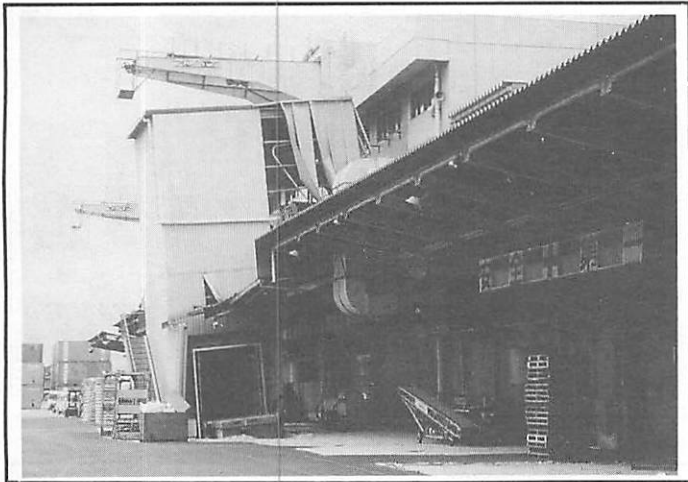
a) Connection Failure of Braced Corrugated Metal Warehouse at Naka Wharf, Port Island
