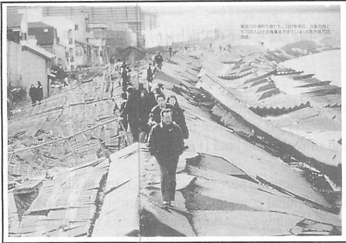
a) Liquefaction-induced Ground Failure along Yodo River (Asahi Newspaper Co., 1995a)
