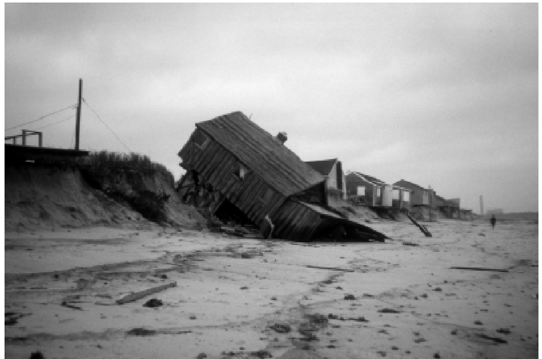
An area of Springhill Beach (Sandwich, MA), where dwellings are at risk due to the episodic storm-induced erosion of coastal dunes.
