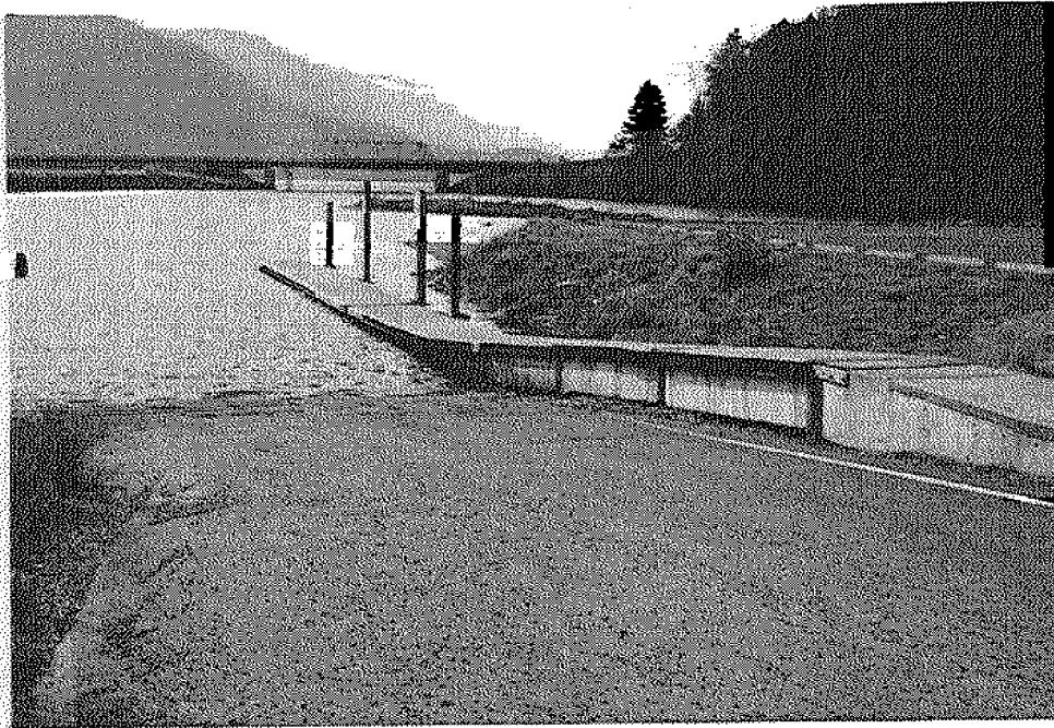
Figure 58 (a): A boating access facility at Wind River. The parking lot is on the right. There are no tie-up devices on the courtesy dock.
