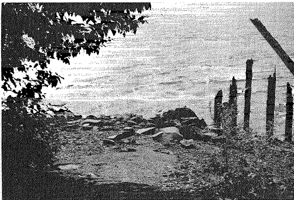
Figure 47: The remains of an old asphalt boat ramp and dock at Fishers Landing at a low water level. The ramp drop-off and large rocks prevent current boating access.
