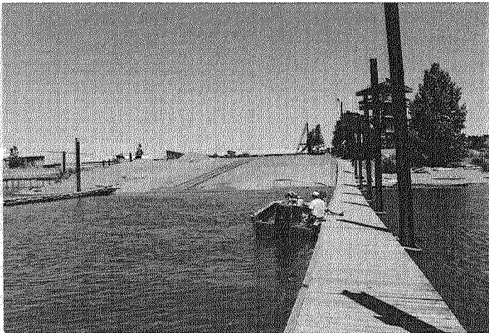
Figure 43 (b): Boating access at Marine Park. The launch ramp is in good condition, but has faded lane markers. The two courtesy docks are in good condition. The viewing platform is on the distant right.
