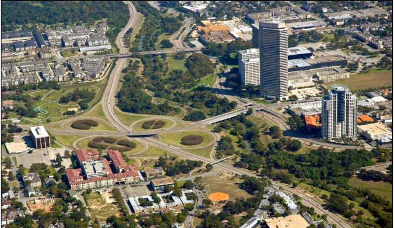
Buffalo Bayou in Houston was modified to some degree, but a natural edge was preserved that provides both aesthetic and functional components, and is in fact iconic of this part of Houston. Incorporating stormwater treatment wetlands into our stormwater detention and conveyance system can add this kind of character to all of our communities. Photo Airborn Imaging.
