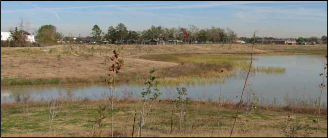
A smooth wetland fringe of bull rushes and other wetland plants adjacent to a side slope at the Willow Waterhole Stormwater Detention Basin in Houston, Texas. The photo was taken during the 2011 drought. Photo courtesy of Harris County Flood Control District.
