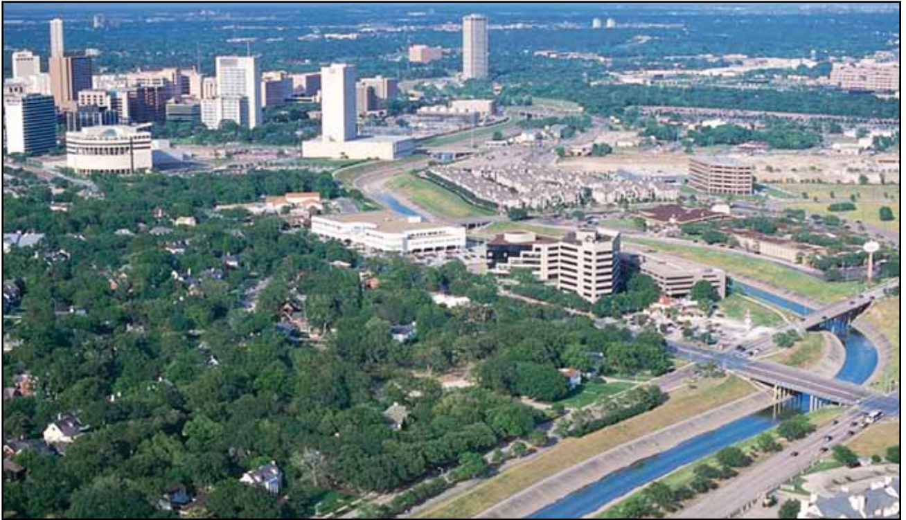
Brays Bayou was once a beautiful coastal stream. Today it serves strictly as stormwater conveyance. This bayou would have to have been modified in any case to accommodate all the new development, but the modification could have included a wider floodplain to accommodate wetlands. Photo courtesy Harris County Flood Control District.
