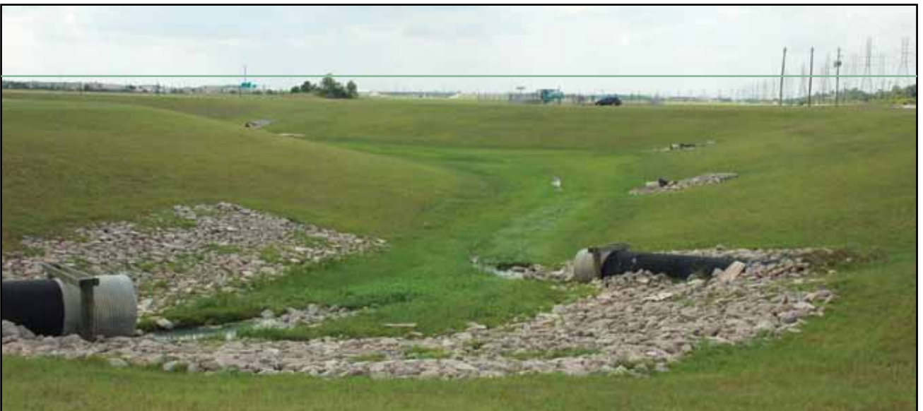
A typical stormwater detention facility, dug deep (more than 20 feet here) to minimize horizontal extent. A wetland capable of treating runoff from the contributing area to this facility would have to be as much as 20-30% larger in horizontal extent. Note that some wetland vegetation is present in the very bottom of this basin. This basin is probably very near the depth of the water table in the area. Photo by John Jacob.
