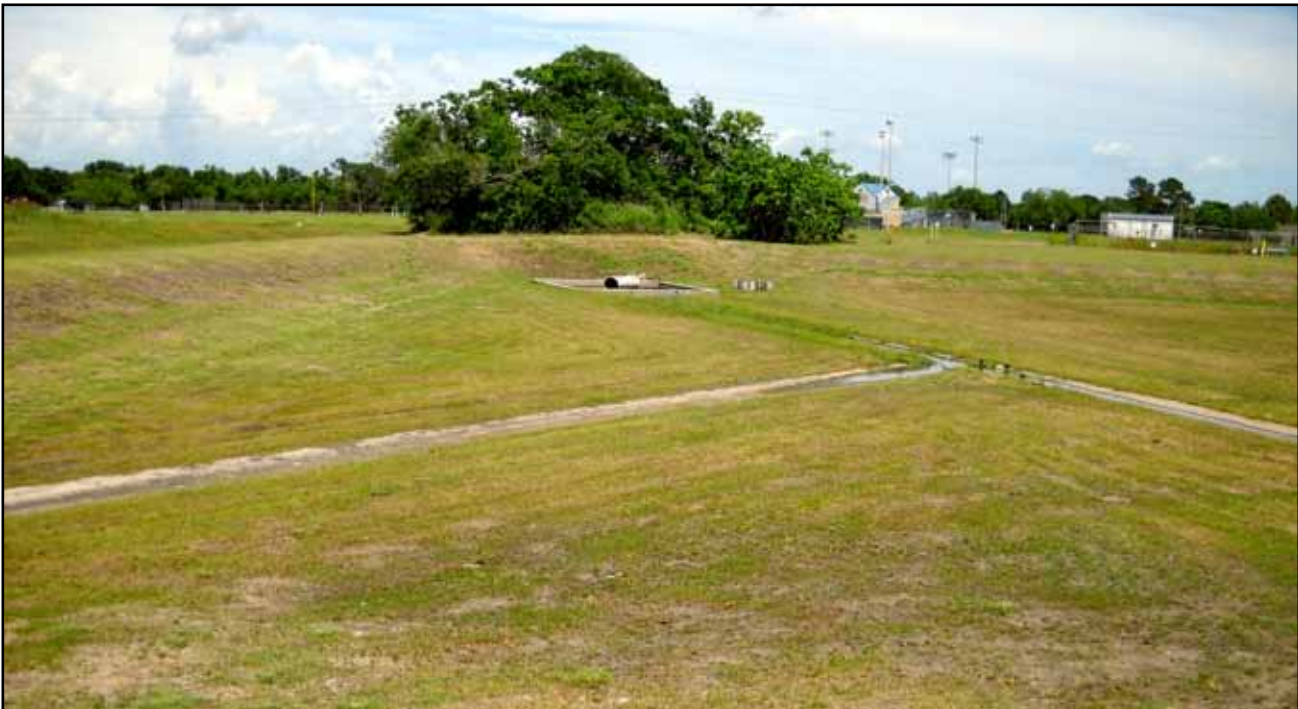
This shallow detention area could easily be configured for a stormwater treatment wetland, transforming an area with little beauty or functionality into a community amenity. Photo by Marissa Sipocz.
