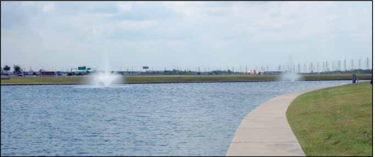
This stormwater detention pond provides some limited stormwater treatment, but it is not a wetland, it does not perform as well as a wetland for water treatment, and it does not have the aesthetic and natural values that a wetland has. Photo by John Jacob.
