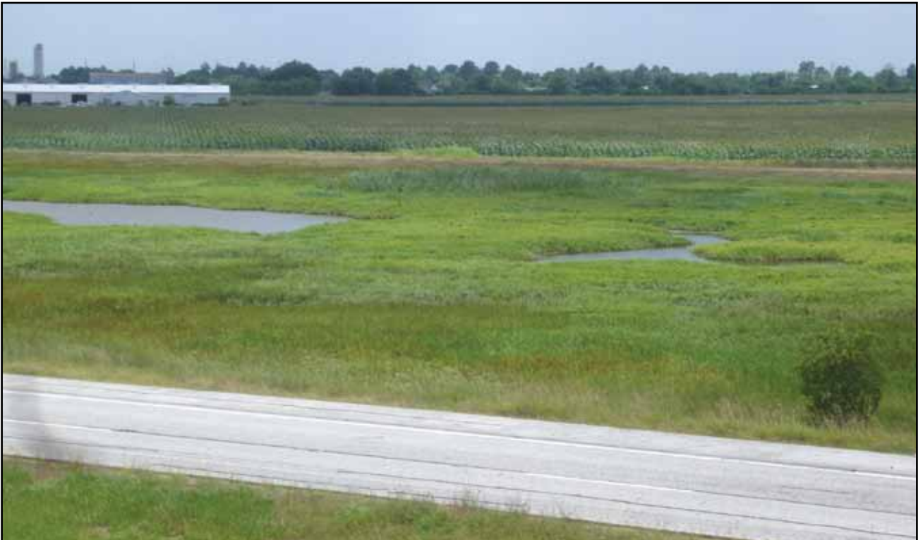
Engineered stormwater wetland at US Hwy 290 and Kickapoo Road, outside of Houston, Texas. This wetland dries out in the summer and is mowed by TXDOT at their regular intervals. Photo by John Jacob.
