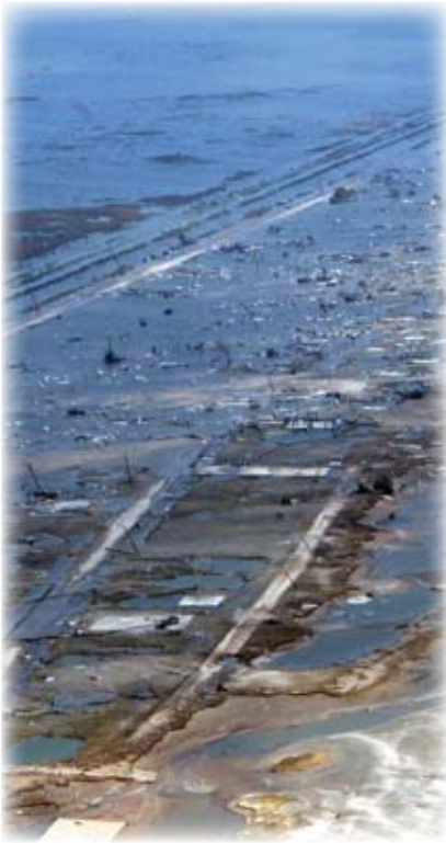
Hurricane Rita devastated Holly Beach, La.
