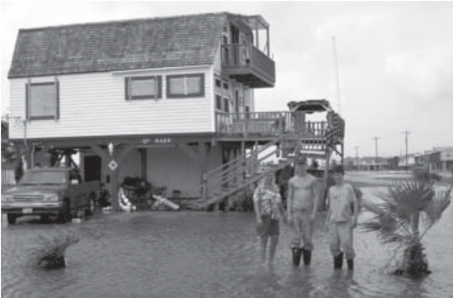
Damage from a Category One hurricane, Claudette, in Surfside, Texas, July 2003.
