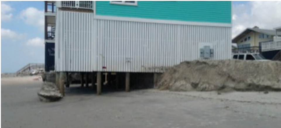
Figure 2. Erosion at Folly Beach caused by Tropical Storm Irene in 2011 and Alberto in 2012, both storms passed more than 100 miles offshore. Photo courtesy of DHEC.
