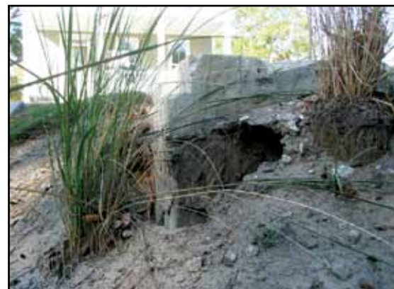
Eroding bioswale
