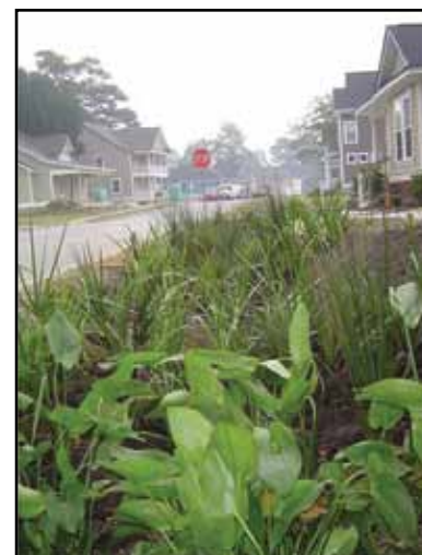
Well-established functioning bioswale
