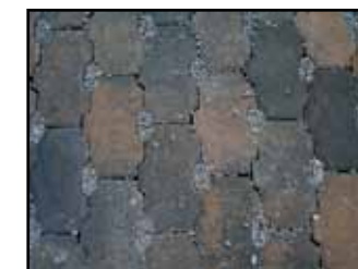
Fully-functional pervious pavers
