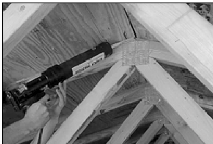
Applying adhesive with standard air powered caulking gun.
