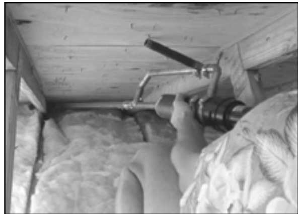
Applying adhesive with the long extension.
