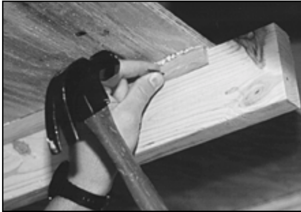
Applying quarter round with adhesive and finishing nails.
