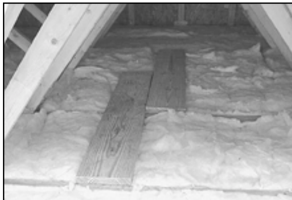
2x10 framing lumber work platform.
