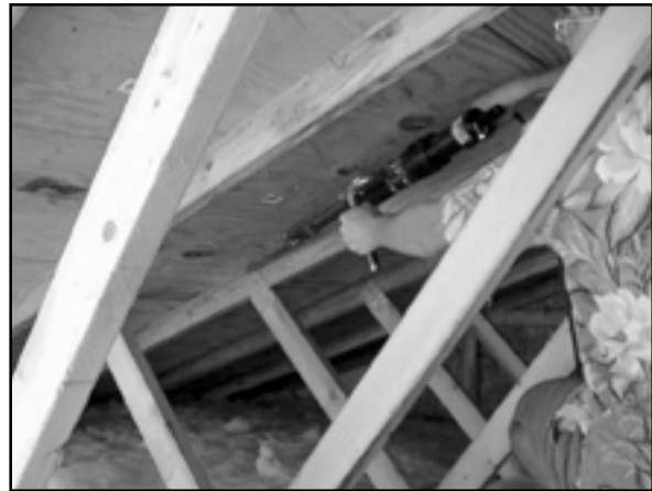
Applying the adhesive with the short extension.
