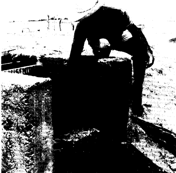
Plate 57. Personnel measuring actual water entering over entrance weir down boards. This exercise is performed in all entrance weirs at two-hour intervals.
