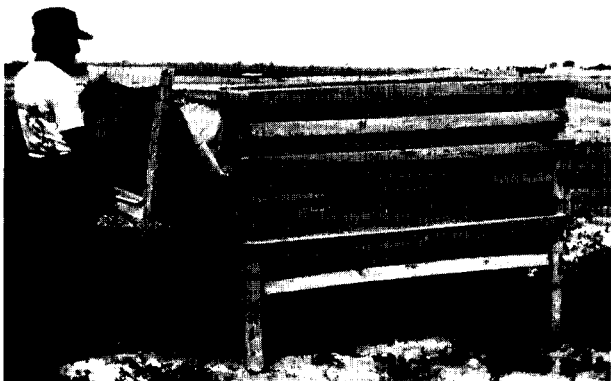
Plate 32. Wooden framed, small mesh harvest box structure that stands partially submerged in harvest basin.
