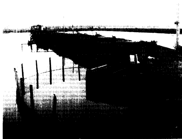
Plate 53. Semi-circular pre-filter screen installed in front of effluent gate to prevent early postlarvae from being forced against screens during strong drainage.
