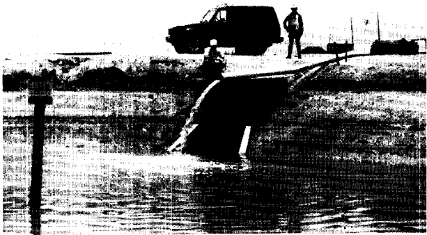
Plate 42. Flushing with fresh water with a 20-cm auxiliary pump to attract juveniles and increase water volume during final transfer procedures.
