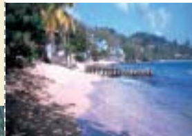
Groynes do not always succeed in promoting sand accretion as seen here at Indian Bay, St Vincent, 1995
