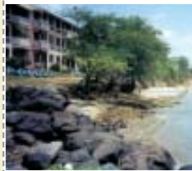
...and erosion on the other side
