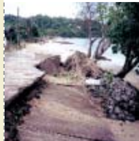
Damage to the coastal road at Havey Vale, Carriacou, resulting from Hurricane Lenny in 1999
