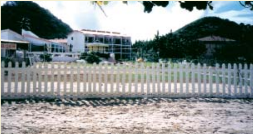
This hotel at Grand Anse, was positioned well behind the dynamic beach area and was safe from Hurricane Lenny's waves, Nov. 1999
