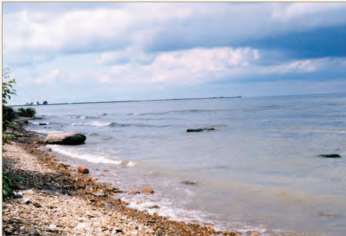
The Conneaut Harbor extends into the lake and interrupts the flow of sediments along the lake shore.
