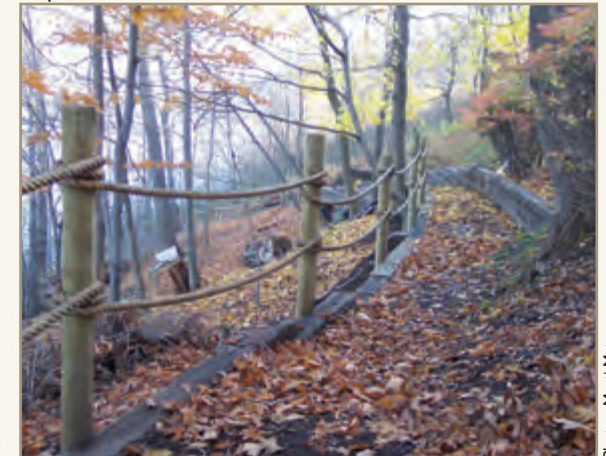
This switchback path was installed to give the homeowners access to the lake with minimal disturbance of the bluff face.
