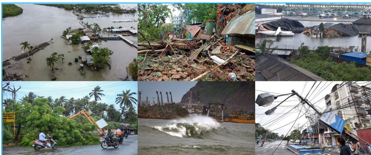
Fig. 4. Damages caused by the Amphan cyclone due to high wind speed and rainfall that affected a large population during 16-23 May, 2020
