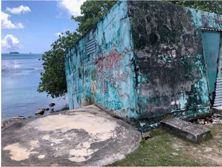
Figure E-5. Cement block structure and associated round cement pad to be demolished. Credit: NMFS, 2021.
