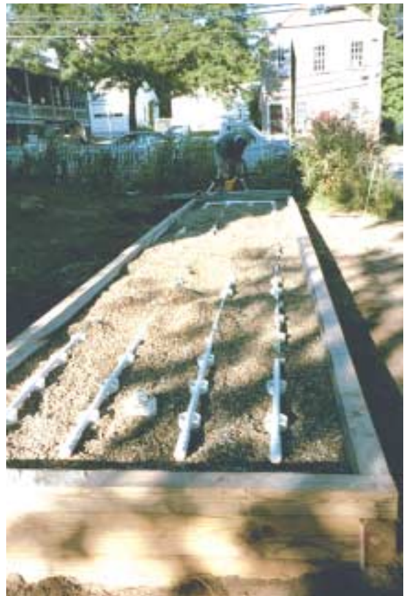
This bottomless sand filter fits into a small space at a property on Main Street.
