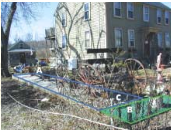
The property owner used plantings and this wagon to disguise the unit's drainfield.
