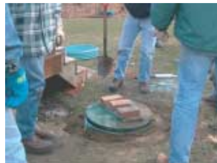
Field workshop for homeowners in septic system maintenance and installation of tank risers, Gloucester, R.I.
