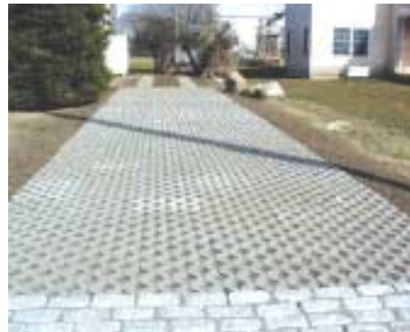
This honeycomb pavement pattern allows for groundwater recharge.
