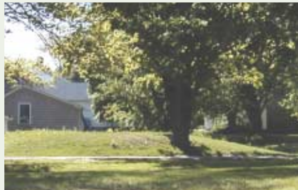
Mound system installed as a repair
