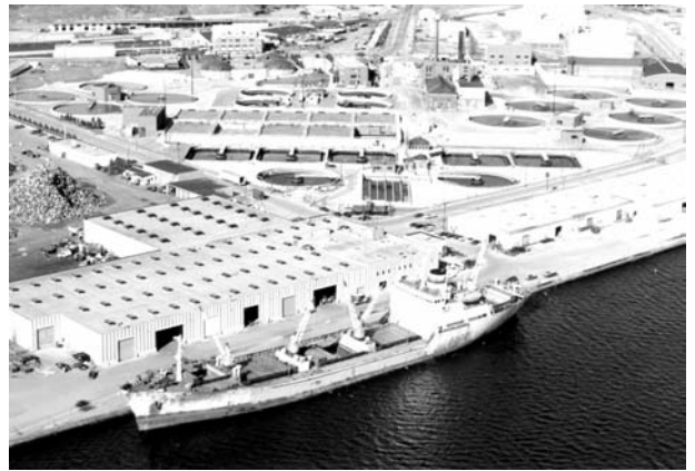
Field's Point treatment facility, Providence, R.I.
