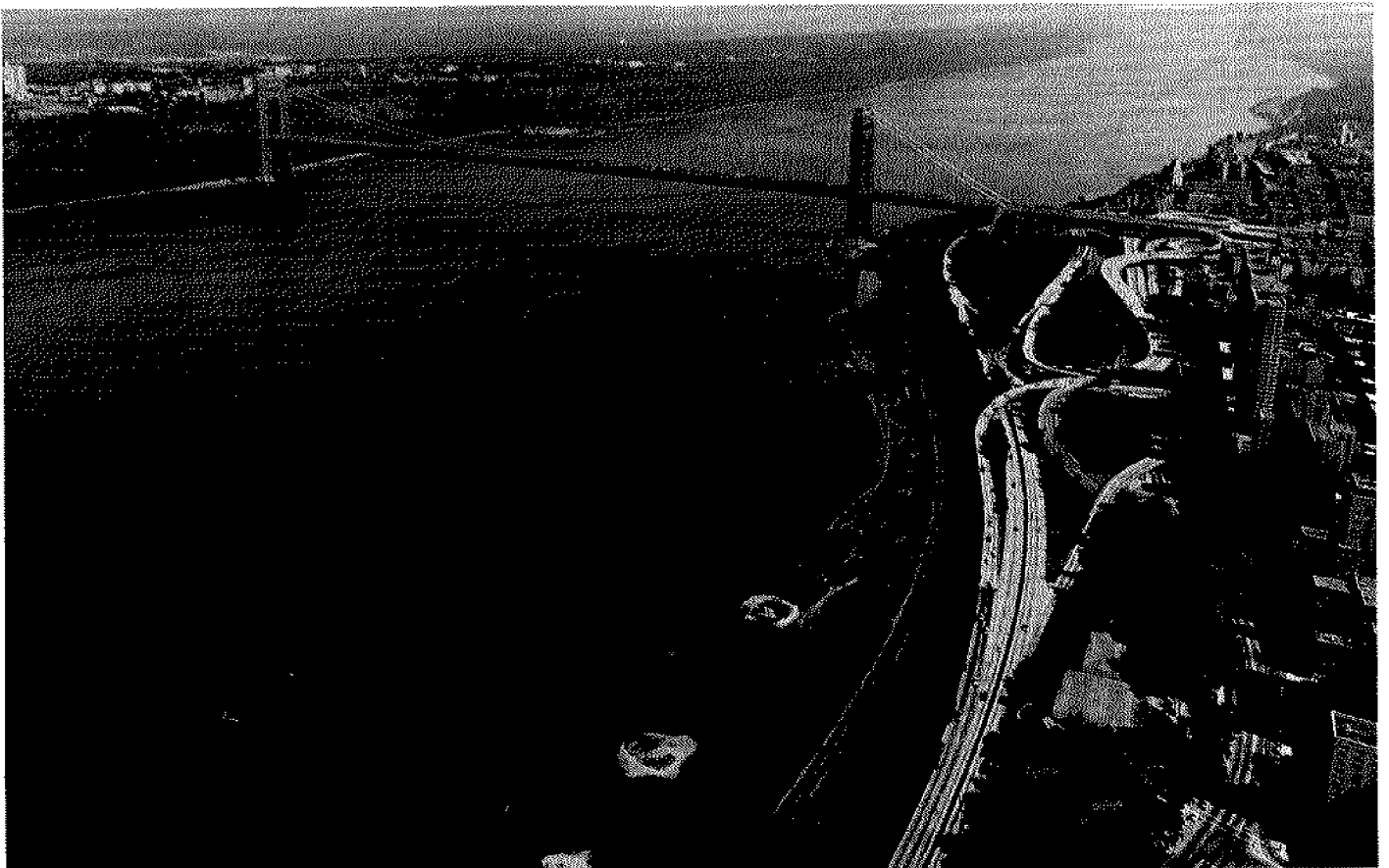
Figure 6. View of George Washington Bridge across Hudson River (Courtesy of Port Authority of New York and New Jersey)
