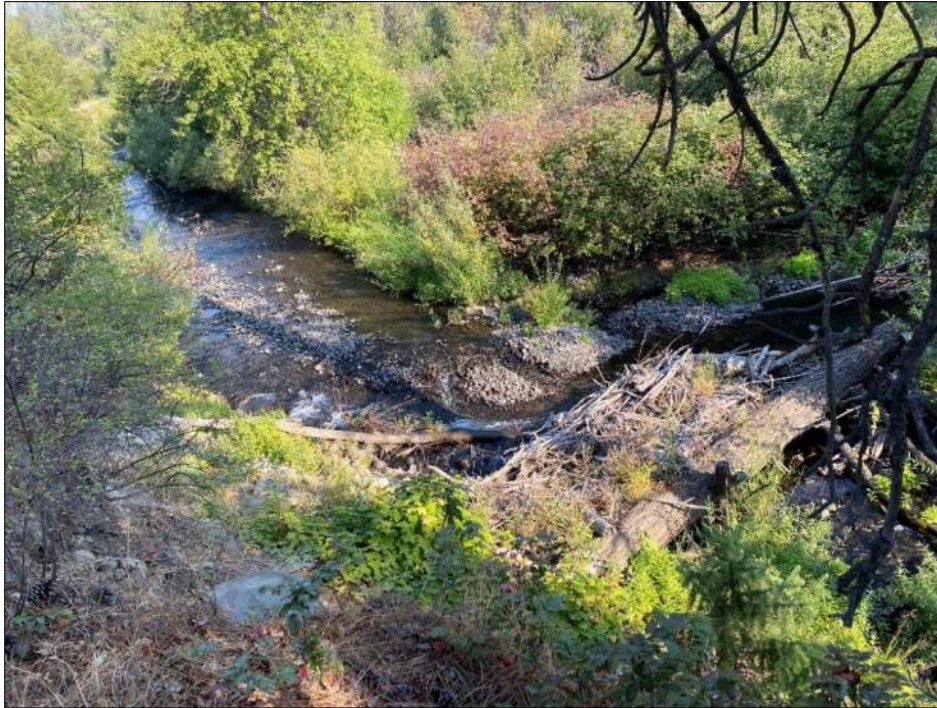
Photograph 7. Channel directly downstream of erosion area, looking north (September 3, 2021).
