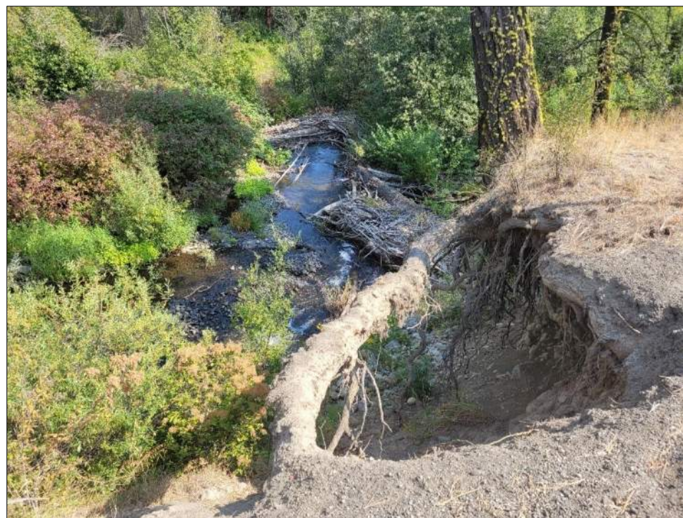
Photograph 2. Above the area of erosion, looking northeast (downstream) (September 3, 2021).
