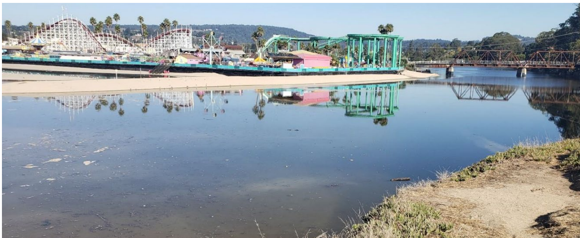
Figure 6. The sand containment berm extension from the corner of the Beach Boardwalk upstream to the railroad trestle bridge. Source: City of Santa Cruz (2021).
