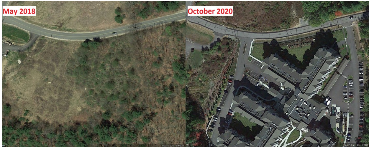
Figure 10. Aerial images of a project area with a CGP NOI stating that there would be “no earth-disturbing activities” (Google Earth)
