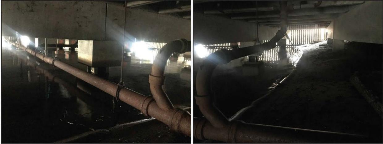
**Figure 4.** Two photographs of the sewer pipe line that is suspended under the Parkside Apartments HOA pier (Adapted Photos 9 & 10 in SUHRCO 2021).
