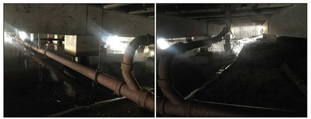
Figure 4. Two photographs of the sewer pipe line that is suspended under the Parkside Apartments HOA pier (Adapted Photos 9 & 10 in SUHRCO 2021).
