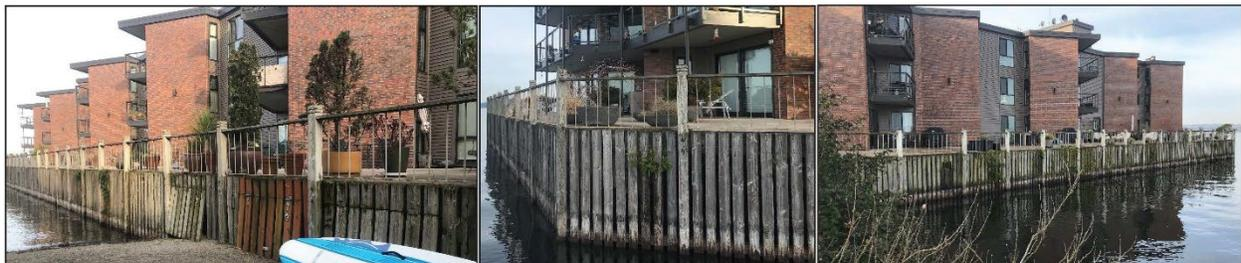
**Figure 3.** Three photographs of the wood skirting and guard rails that surround the perimeter of the Parkside Apartments HOA pier (Adapted Photos 1, 3, & 4 in SUHRCO 2021).
