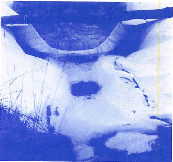
Low cost plastic dam for herring runs, a joint M.I.T.-U.Mass. Sea Grant project.
