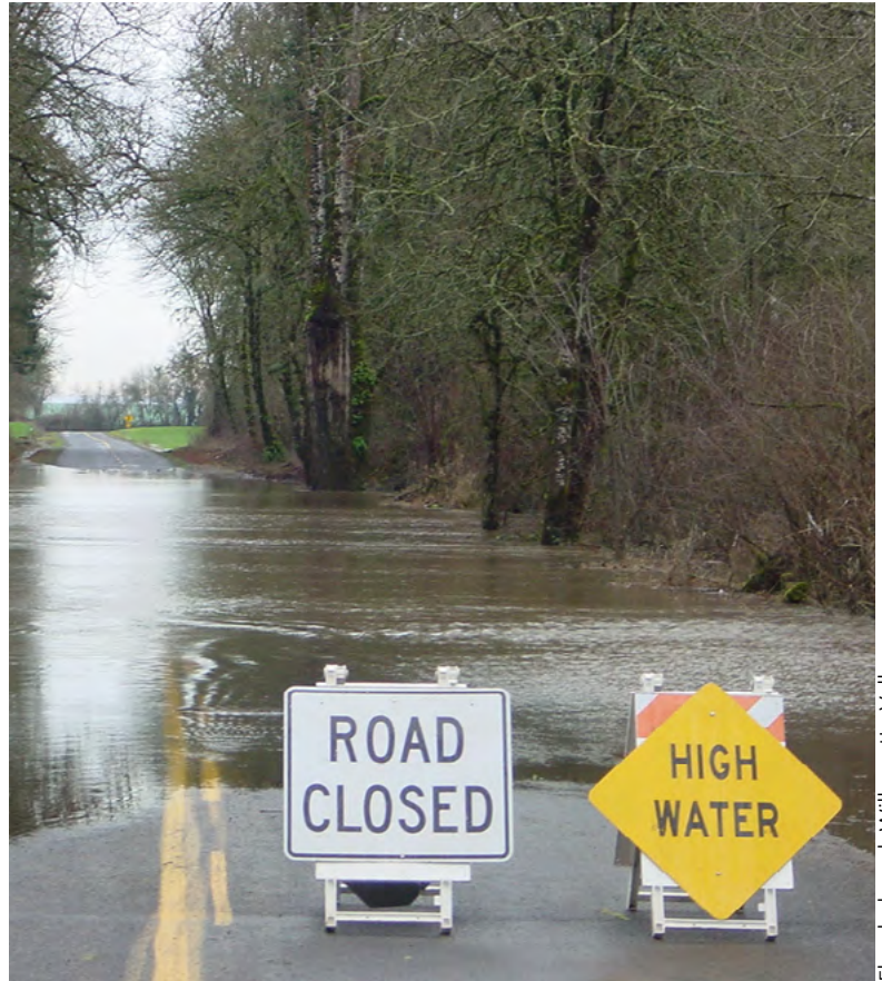
Flooded road, Willamette Valley
