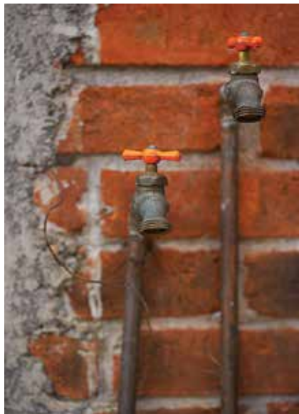
Nearly all of the system managers interviewed perceived their drinking water system infrastructure as a major risk.
