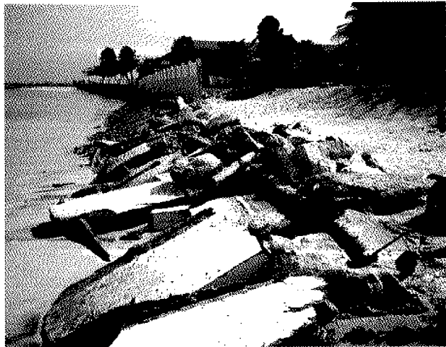
Photograph 2. Eroded beach, Runaway Bay, Antigua, 1997. Erosion of the sand has caused walls to collapse leaving concrete debris on the beach as the land edge retreats inland.
