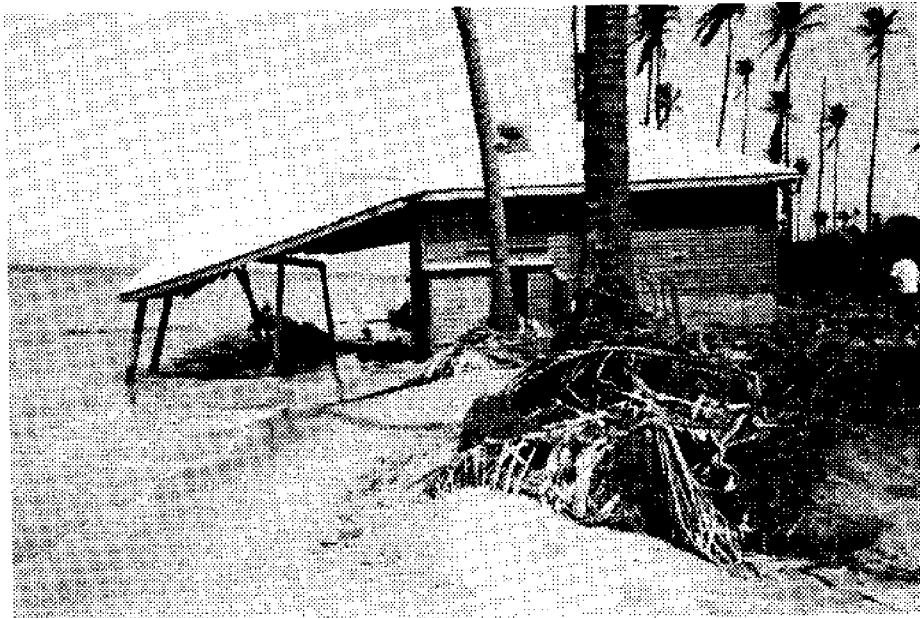
This restaurant is a victim of coastline retreat. Construction setbacks should take adequate account of such potential encroachment of the sea.
