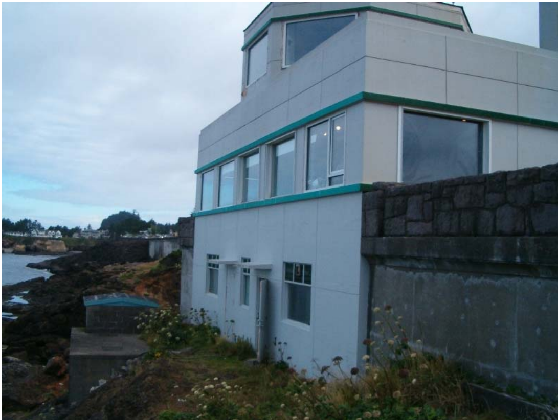
Figure 2. Overview of Whale Watch Center seaward side from the south.
