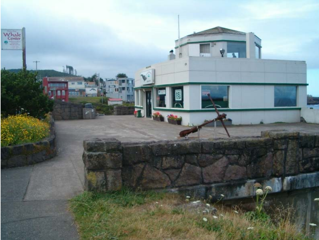
Figure 3. Overview of Whale Watch Center from the north showing primary entrance on second level, upper viewing deck, and landscape features.
