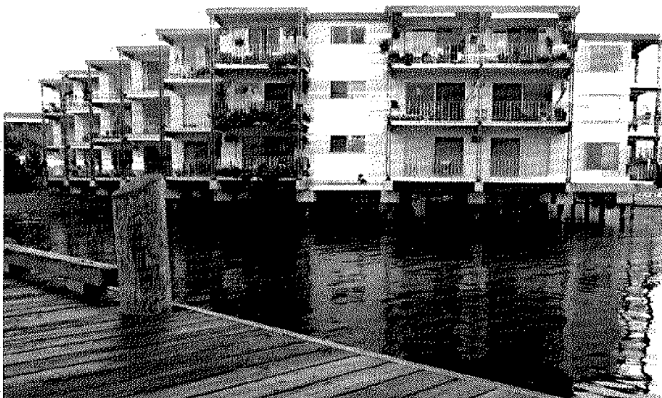
Revitalization efforts in Kirkland, Washington, had to contend with existing residences.
