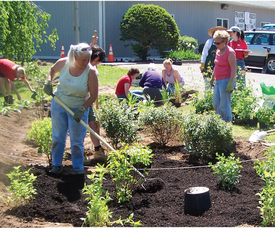
400 square foot garden installed at the town of Saugerties Senior Citizen Center to catch run off from the building and parking lot.
