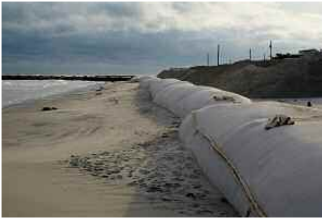
Figure 11. Exposed geotube after Superstorm Sandy in Ocean City, New Jersey.
