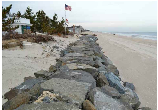
Figure 13. Exposed dune rock core after Superstorm Sandy in Bay Head, New Jersey.
