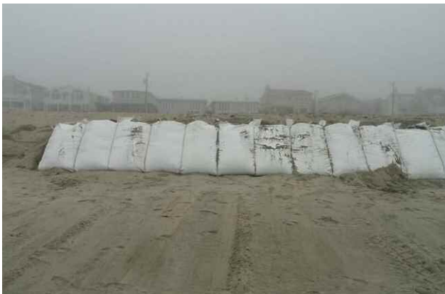
Figure 12. Trapbag geotextile (geocube) container installation in Ocean City.
