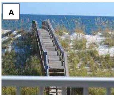
Figure 16A. Wooden dune walkover (preferred method); B. angled walkway through dune; C. shore-perpendicular walkway through dune (least preferred method).
