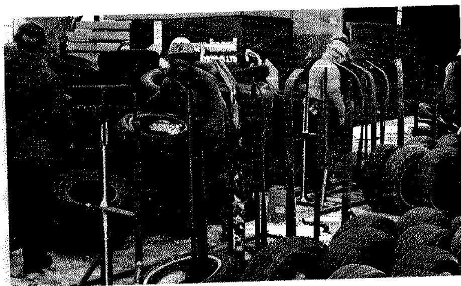
Figure 15. Tire frames used to assemble Goodyear FTB modules. (Bishop and Gallant 1981)
