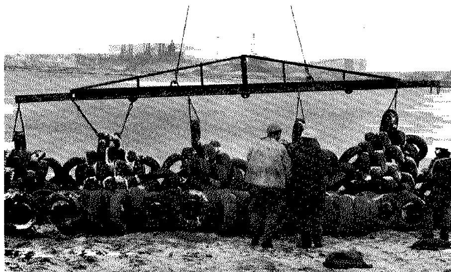
Figure 18. Row of 9-module-wide Goodyear FTB is lifted into the water. (Bishop and Gallant 1981)
