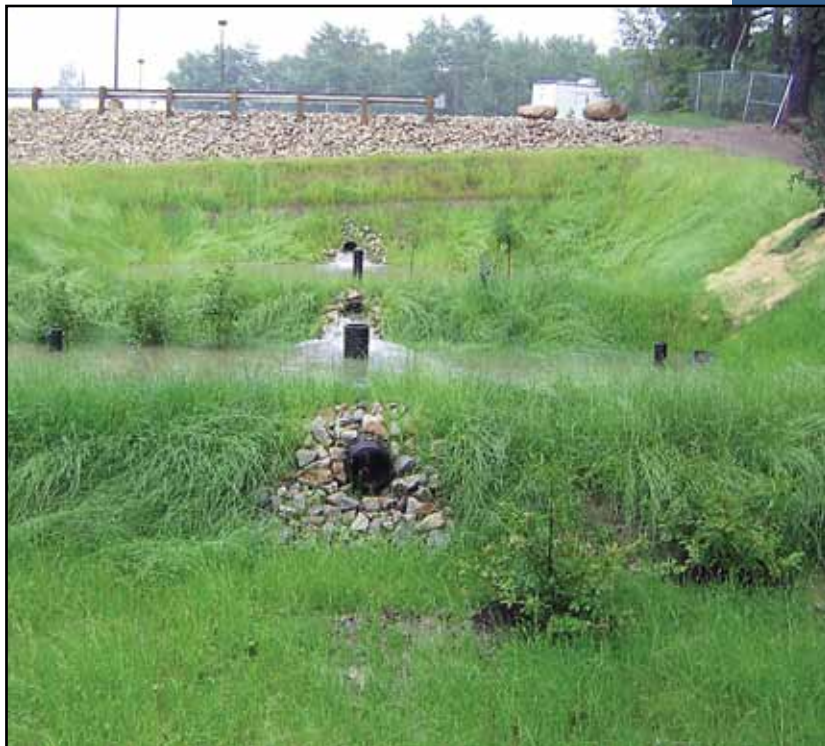
Gravel wetland operation in a rain event.
