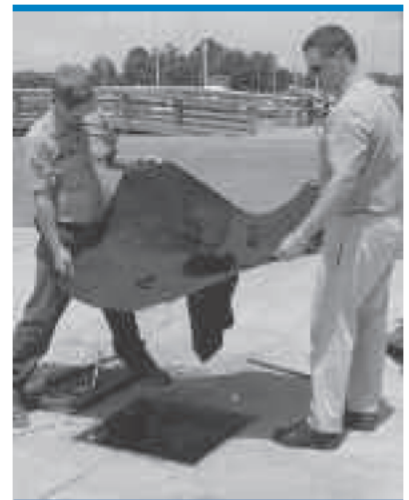
Inlet filter sock being installed.
