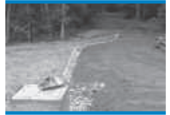
Level spreader constructed of concrete.
