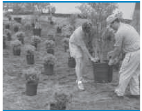
Installation of plants in a rain garden at Carolina Beach State Park Marina.
