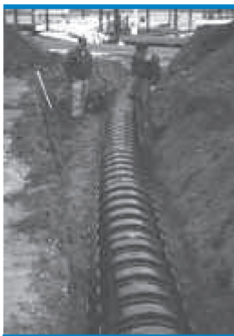
Infiltration chambers being installed.
